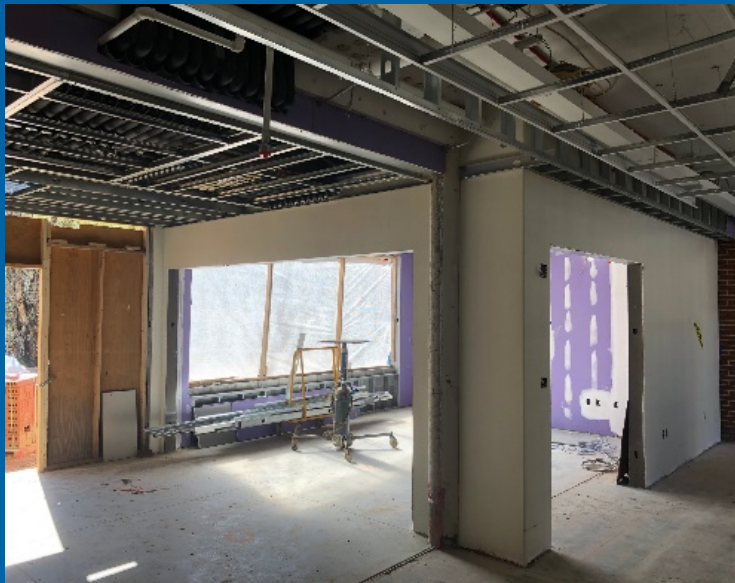
Main Entrance Drywall and Framing
